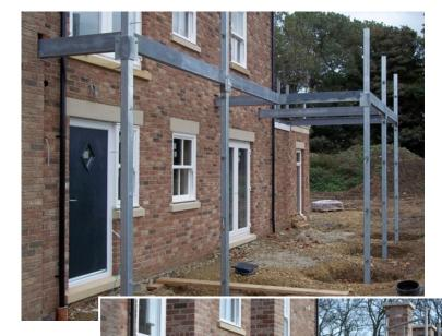
**BEFORE** - Balcony Support Steelwork - Private Residence in Middlesbrough AFTER - Bricked-Up and Timber Decking Supports Installed
