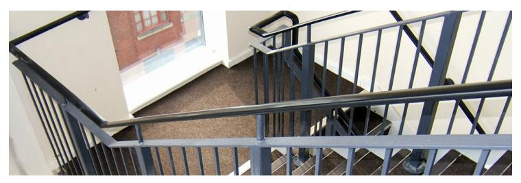
We offer two basic mild steel balustrade designs which are appropriate for both top-fixing and side-fixing. Matching wall mounted handrail is supplied for all of our balustrade designs.
