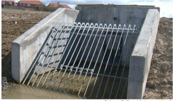
Culvert Grille with Access Hatch
