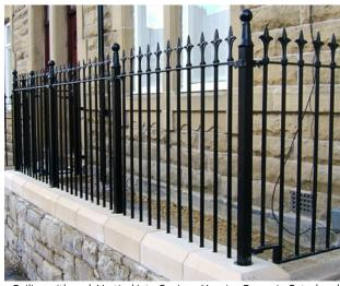
Railing with each Vertical into Coping - Housing Regen in Gateshead
