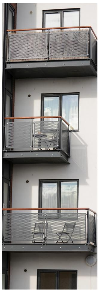
Perforated Plate & Timber Rail Balconies - Housing in Middlesbrough
