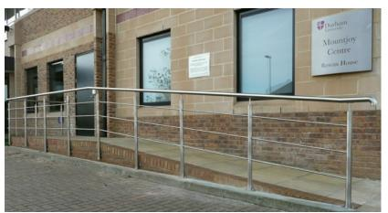
External Solid Bar Infill Balustrade - DDA Works in Durham
