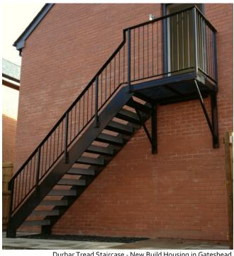
Durbar Tread Staircase - New Build Housing in Gateshead
