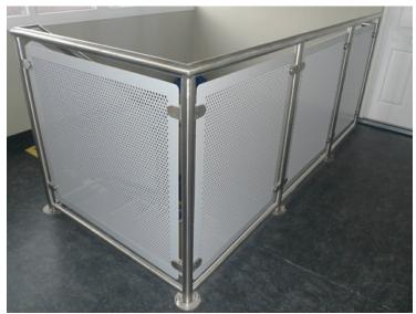
Perforated Plate Internal Balustrade - Housing Regeneration in Stockton
