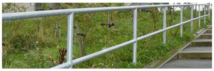
Tubular balustrade is generally used externally to offer support for pedestrians using stairs, ramps or pathways. It is also used to protect the public from hazards.
