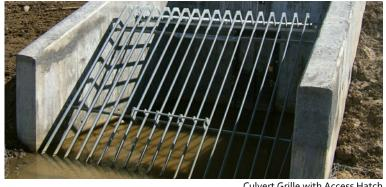
Culvert Grille with Access Hatch
