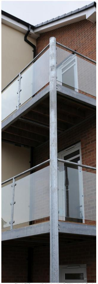
Glass Infill Structural Balconies - New Build Housing in Cleadon
